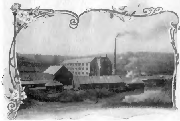
BRIMSCOMBE UPPER MILLS. (P. C. Evans & Sons).
