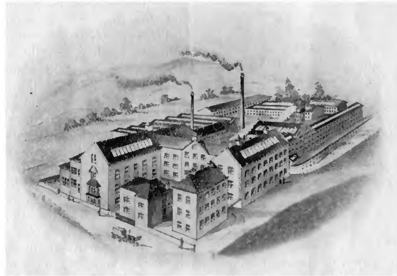
VIEW OF DUDBRIDGE MILLS, STROUD. (Apperly, Curtis & Co., Ltd.)
