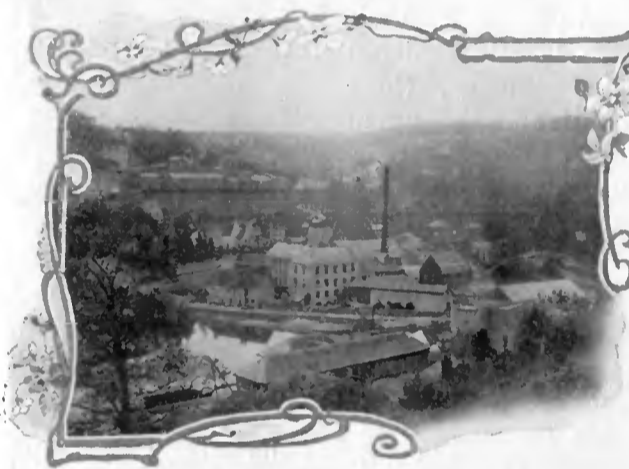
BRIMSCOMBE PORT MILLS. (P. C. Evans & Sons).
