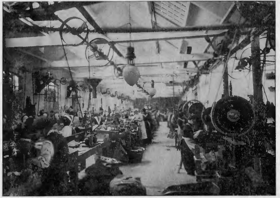
AN INTERIOR VIEW, STROUD METAL COMPANY'S WORKS.
