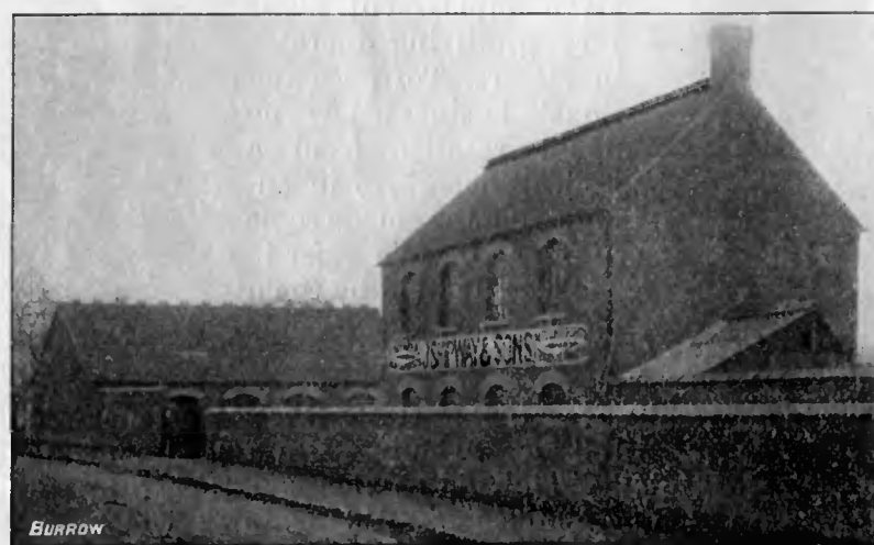
EBLEY IRON WORKS, STROUD. (Jehu Shipway & Sons.)
